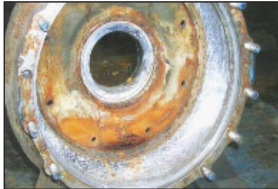
Condition of pump after 9 months
